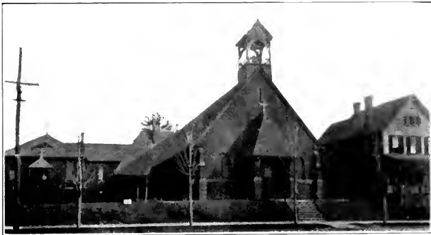
CHURCH OF THE HOLY CROSS, (Episcopalian).
